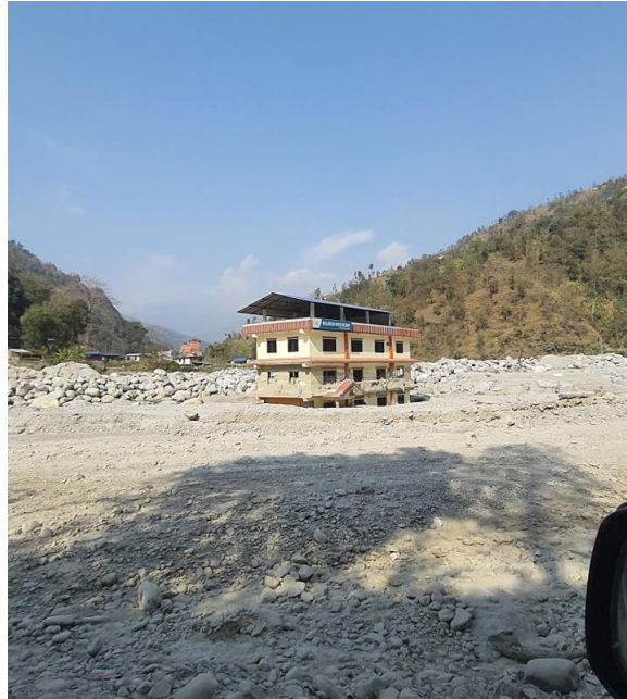
Destruction at Melamchi area from upstream landslide
