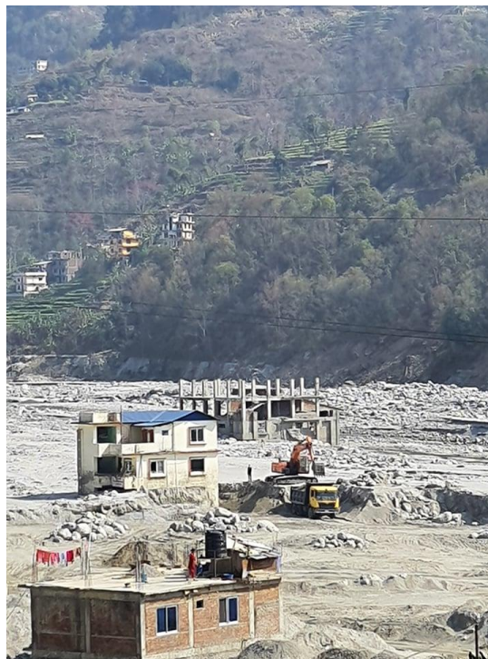
Damage devastating landslide and flood at Indrawati area from upstream landslide
